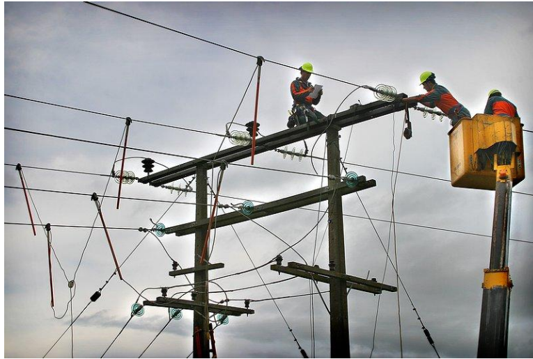
Photo 1 - Staff undertaking maintenance on 33kV line
