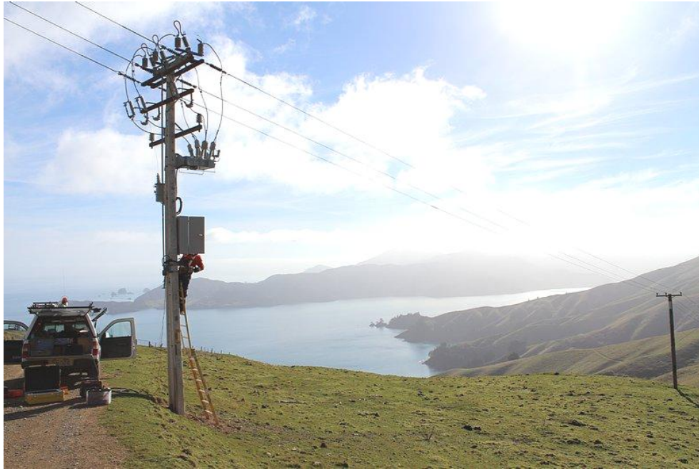
Photo 5 - testing new recloser, Saddle Hill
