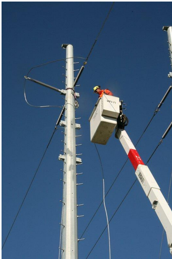
Photo 21 - 33kV line renewal
