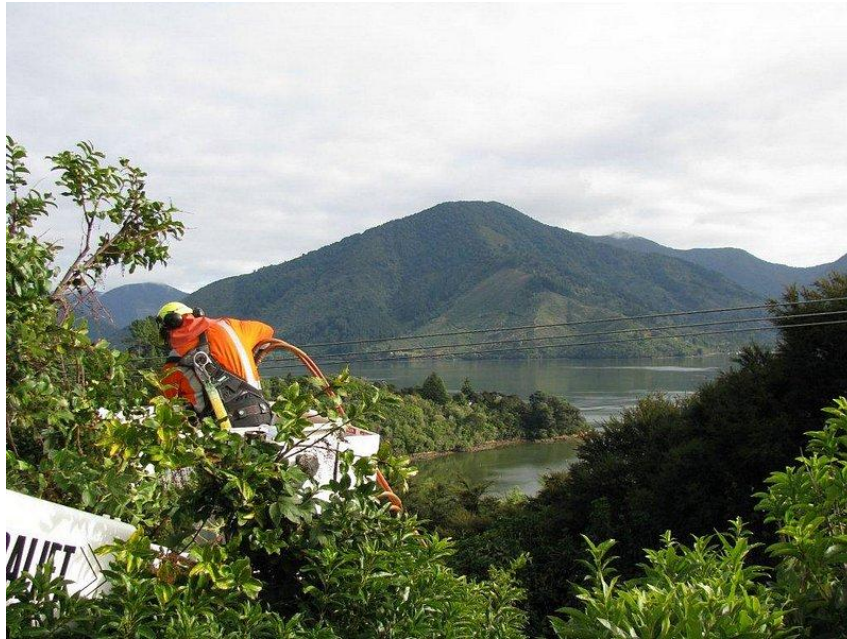
Photo 16 – Trimming Vegetation near 11kV line
