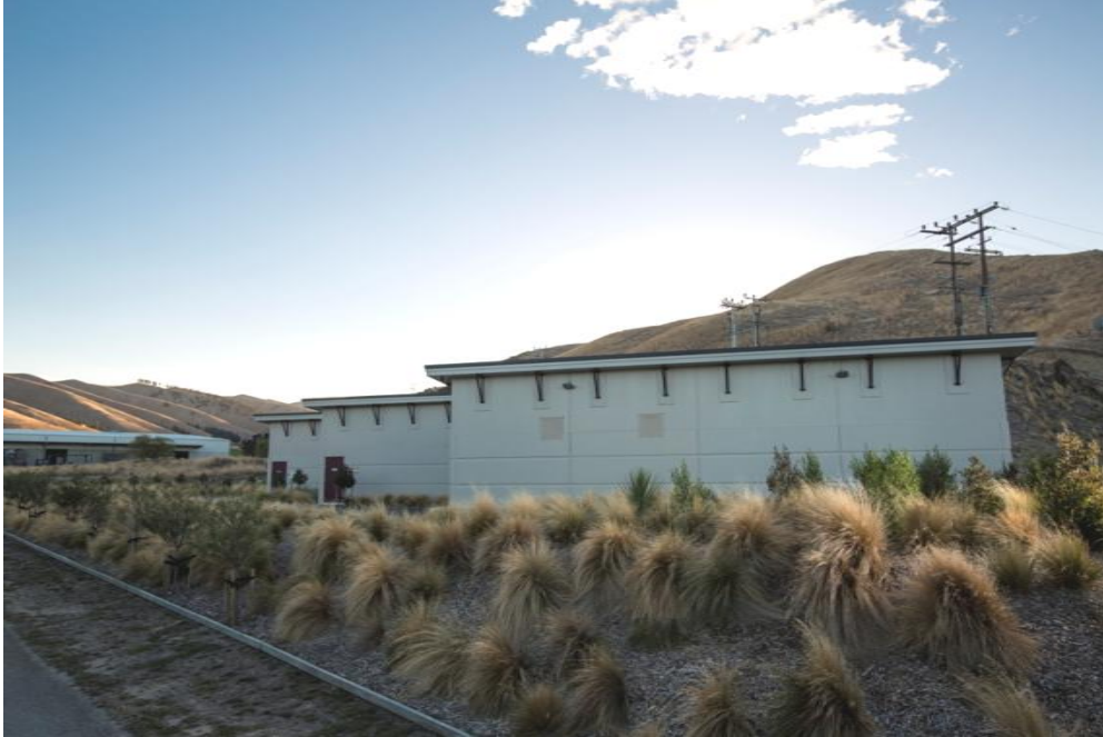
Photo 20 – Cloudy Bay Substation
