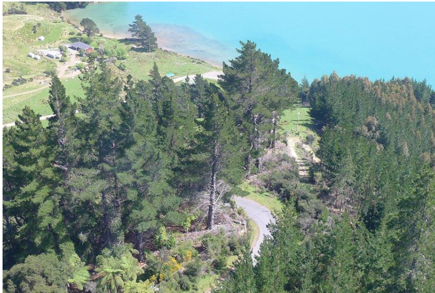
Photo 6 - 11kV line through Trees
