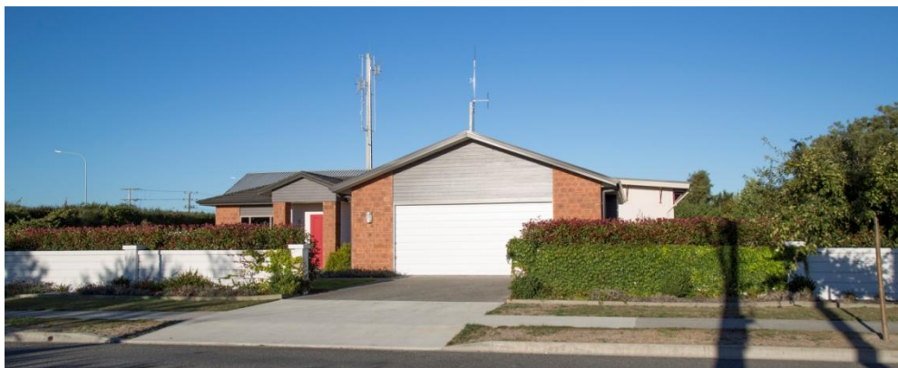
Photo 18 – Springlands substation, Blenheim
