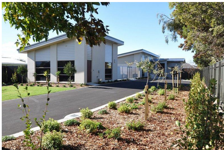
Photo 8 - Waters Substation, Blenheim
