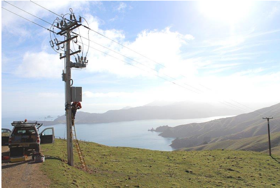
Photo 5 - testing new recloser, Saddle Hill
