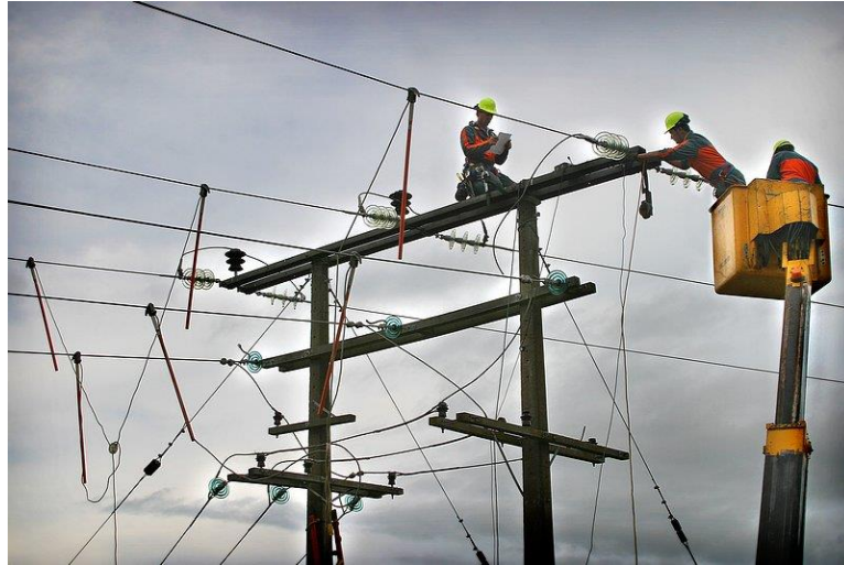
Photo 1 - Staff undertaking maintenance on 33kV line
