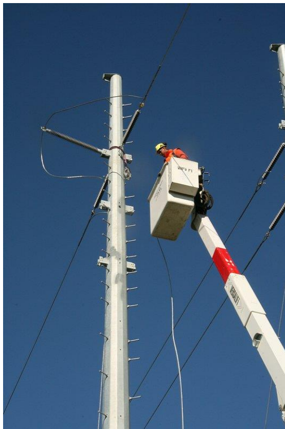
Photo 19 - Maintenance work being undertaken on steel pole components
