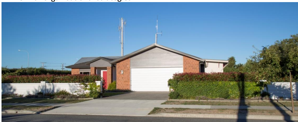
Photo 16 - Springlands Substation, Blenheim
