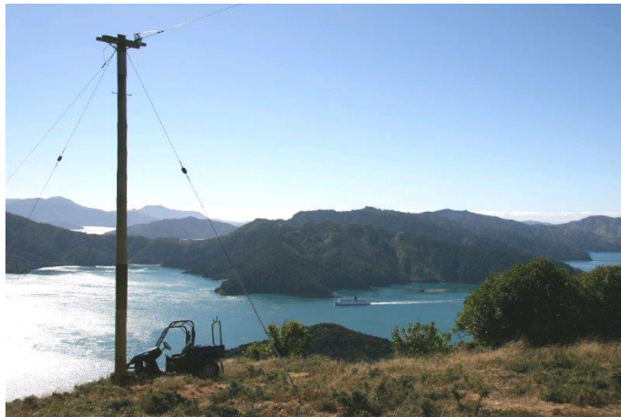
Photo 11 - SWER lines in Tory Channel
