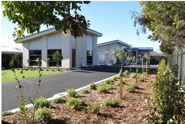
Photo 8 - Waters Substation, Blenheim
