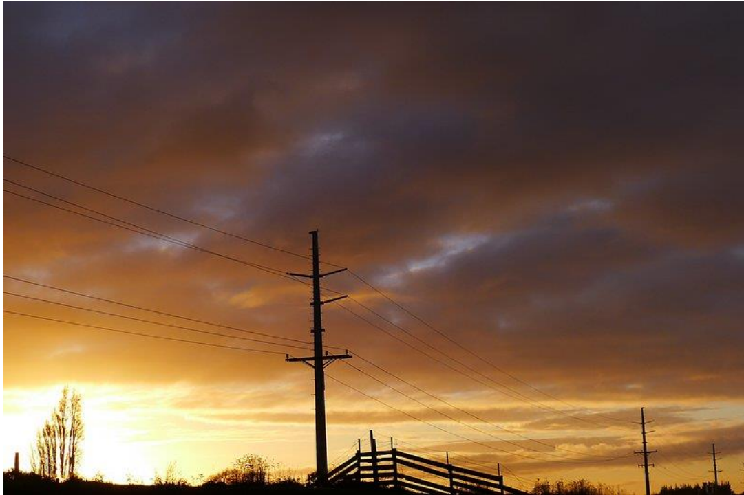
Photo 2 - renewed 33kV Line Landsowne Park to Riverlands - Steel Poles
