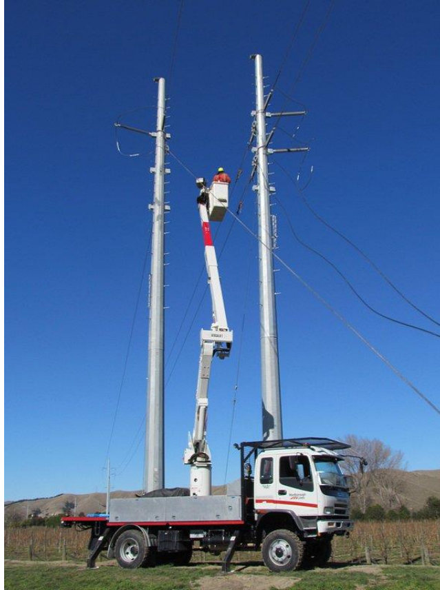
Photo 14 - Work on Renewal of Lansdowne to Riverlands 33kV line
