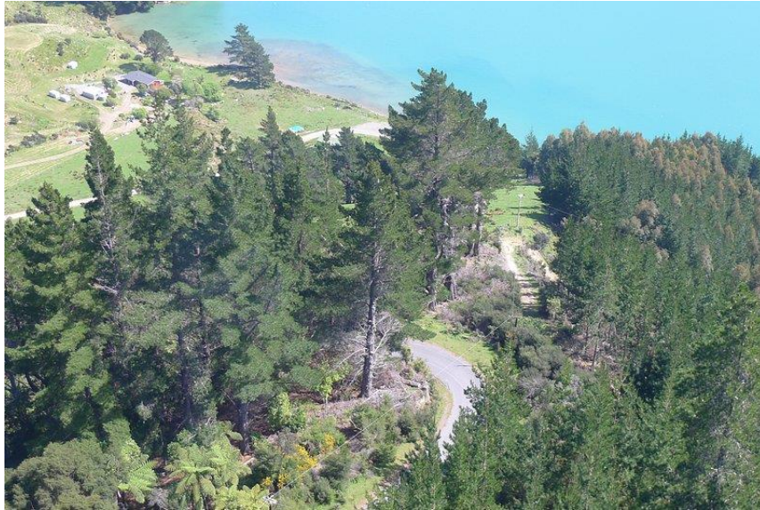
Photo 6 - 11kV line through trees
