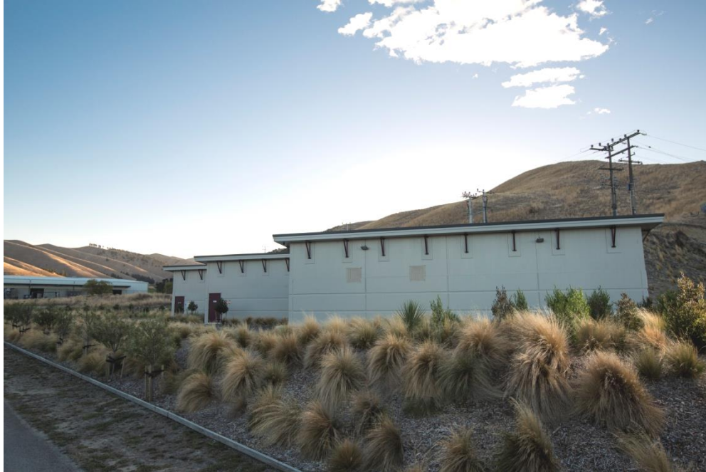
Photo 18 - Cloudy Bay Substation
