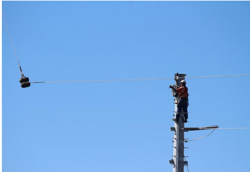
Photo 10 - Lineman placing rope from helicopter into pulley line roller
