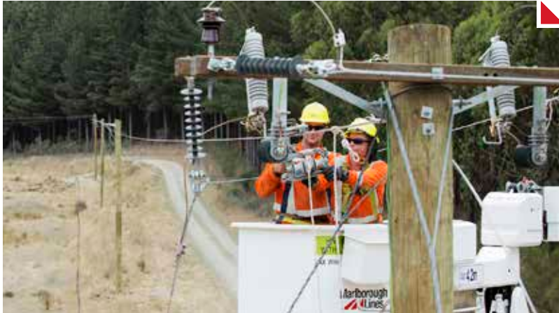
1 Linemen creating a new catenary insulated line on a forest margin.
