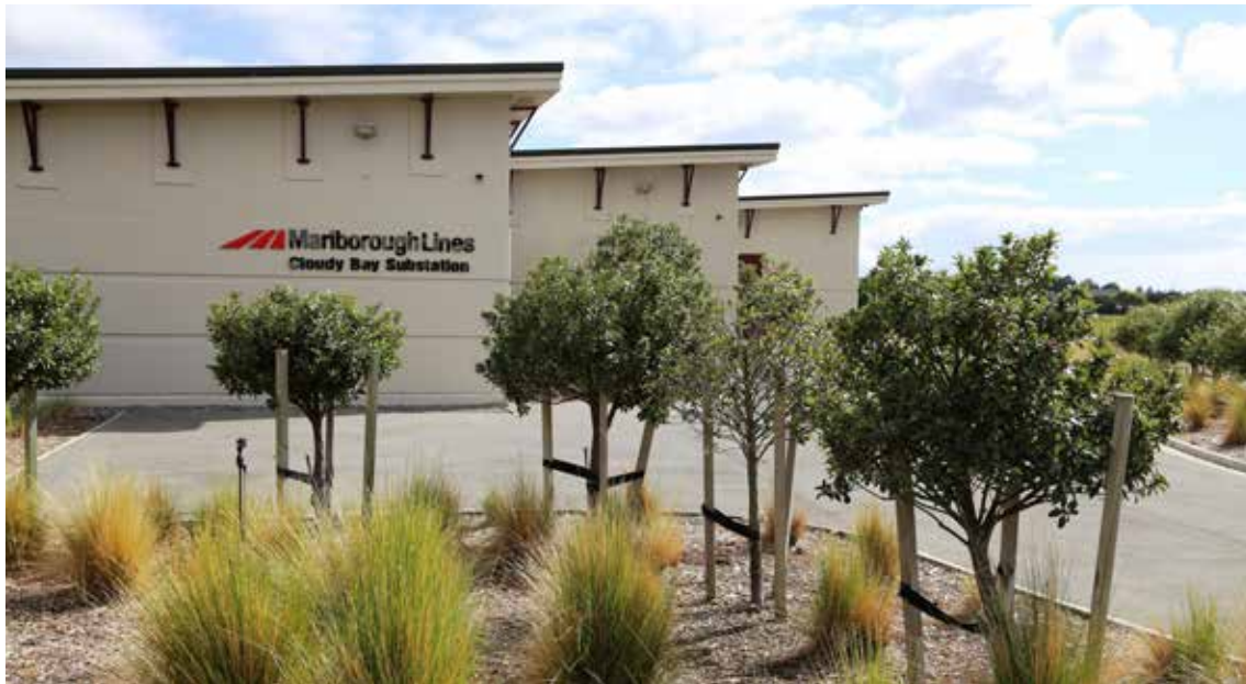
Our larger zone substations are attractively landscaped and with zero noise emissions they make great neighbours.
