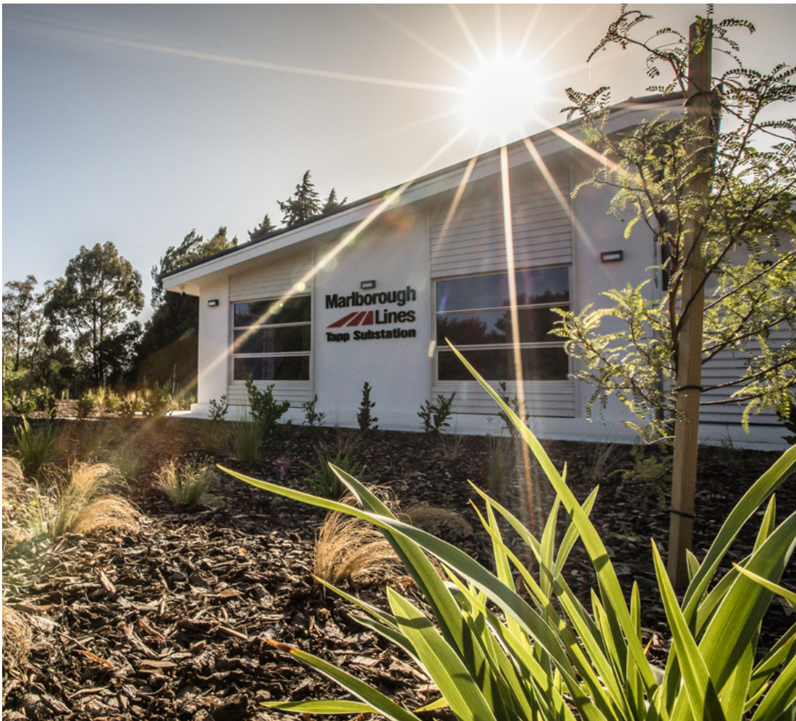
Tapp Substation located in Renwick is our latest indoor zone substation which integrates into the suburban surrounds and has been extensively landscaped to blend into the local environment.
